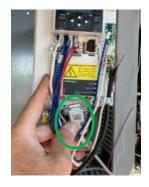
5) Then disconnect the CAN U600X cable on the side of the CCL terminal strip
