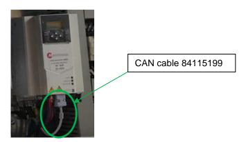
12) Connect the Can cable, code 84115199, to the CCL terminal strip.
